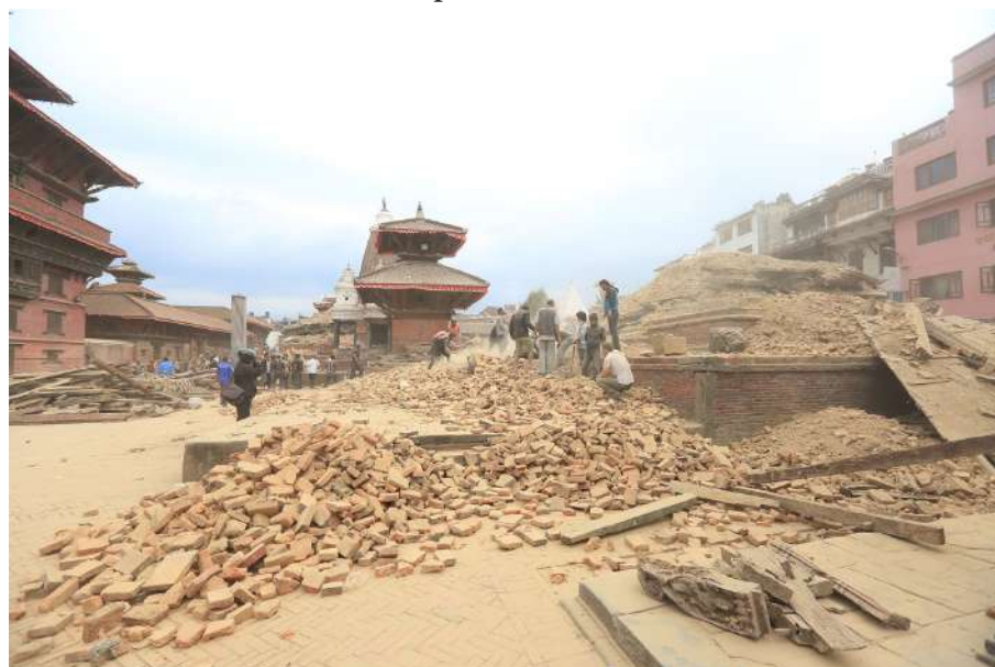
Photo 2: “Gorkha” Earthquake Damage in Kathmandu Valley (UNDP, 2015)
